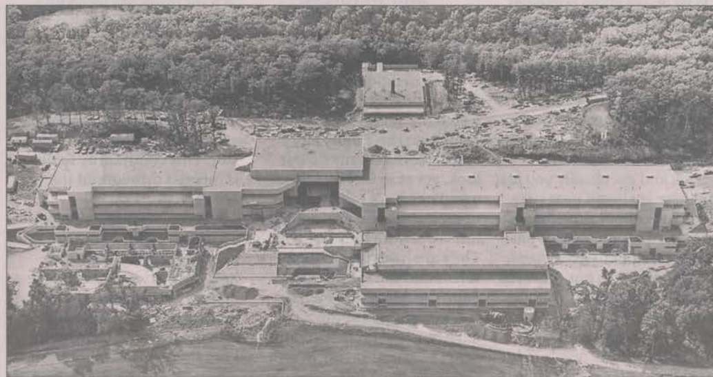
A Sept. 13, 1973 aerial view of the new Holyoke Community College on Homestead Avenue shows a modified "megastructure" consisting of a compact group of buildings built in tiers on a natural ridge. (REPUBLICAN FILE PHOTO)
